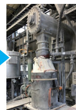
Filled into flexible container bags
