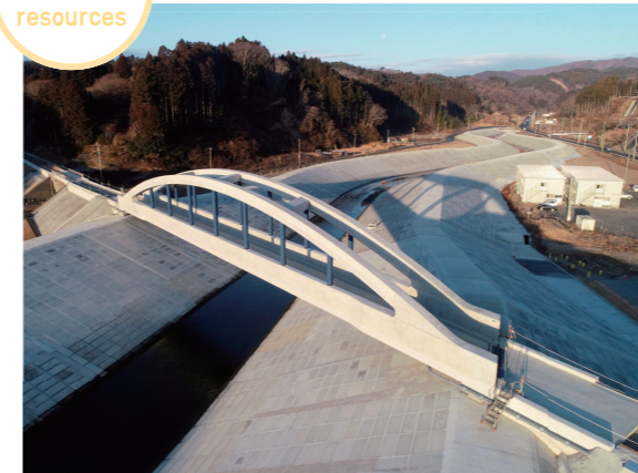
JR Kesenuma Line Sakuragawa Bridge (Minamisanriku-cho, Miyagi Prefecture) (CFFA® used for bridge girders, arches, and longitudinal steel)
